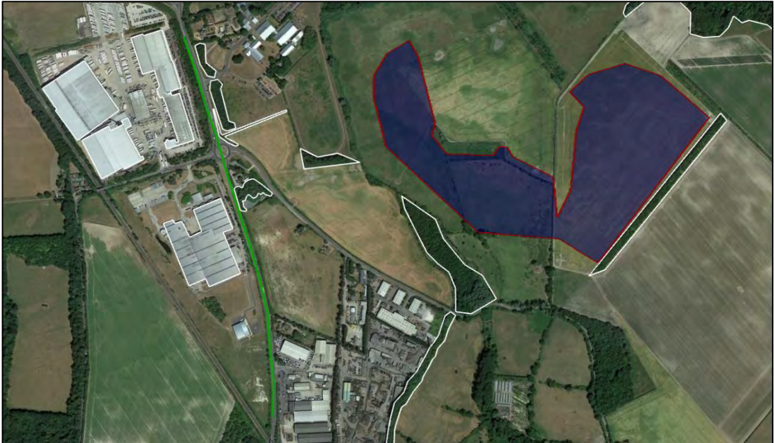
Figure 16 Post mitigation effects towards the A142
